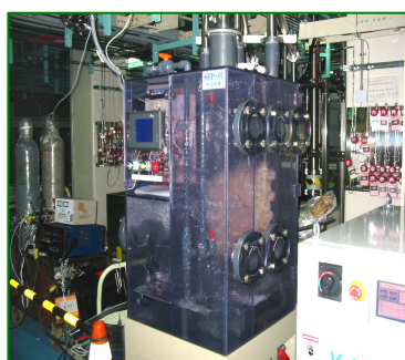
▲ Waste gases are first treated at local scrubbers inside the fab, then at central scrubbers, and finally exhausted
