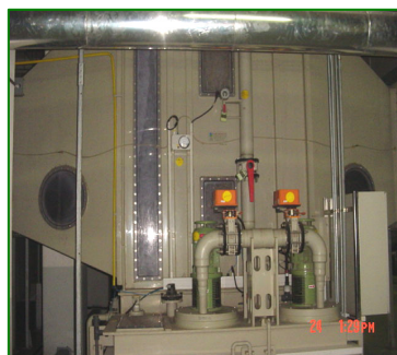
▲ Waste gases are first treated at local scrubbers inside the fab, then at central scrubbers, and finally exhausted
