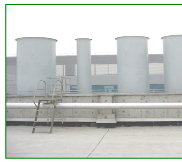
▲ Waste gases are first treated at local scrubbers inside the fab, then at central scrubbers, and finally exhausted
