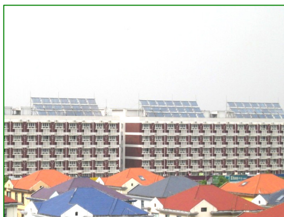
▲ Solar thermal water heaters on top of the dormitories
