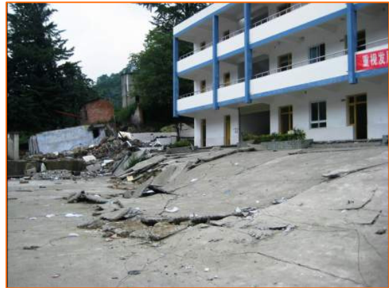
▲ Cracked concrete in pavement in a courtyard
