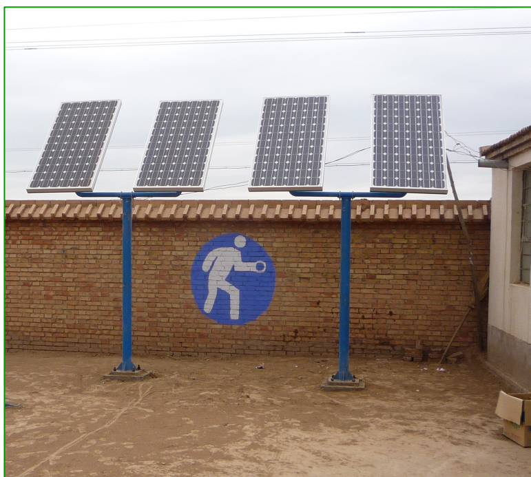
▲ Donated solar panels installed at a school in Ningxia
